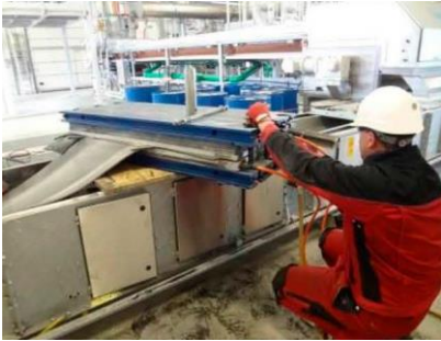
Hot splice with Multiface.
