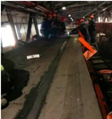
Repair of long breaks.
